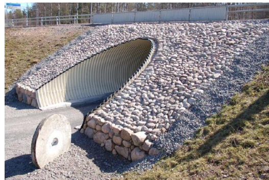
Foto 4. Betoonalusel munakividega kindlustamine (foto: Sten-Eric Lager [29])
